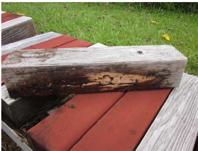
Figure III-5. Example of a non-treated Douglas-fir crossarm section with visible decay after 4 years of exposure in Hilo, Hawaii.
