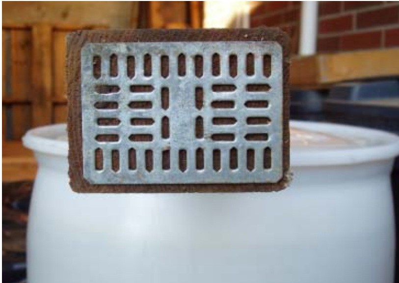
Figure III-9. Example of an end-plate on a penta treated Douglas-fir cross arm.
