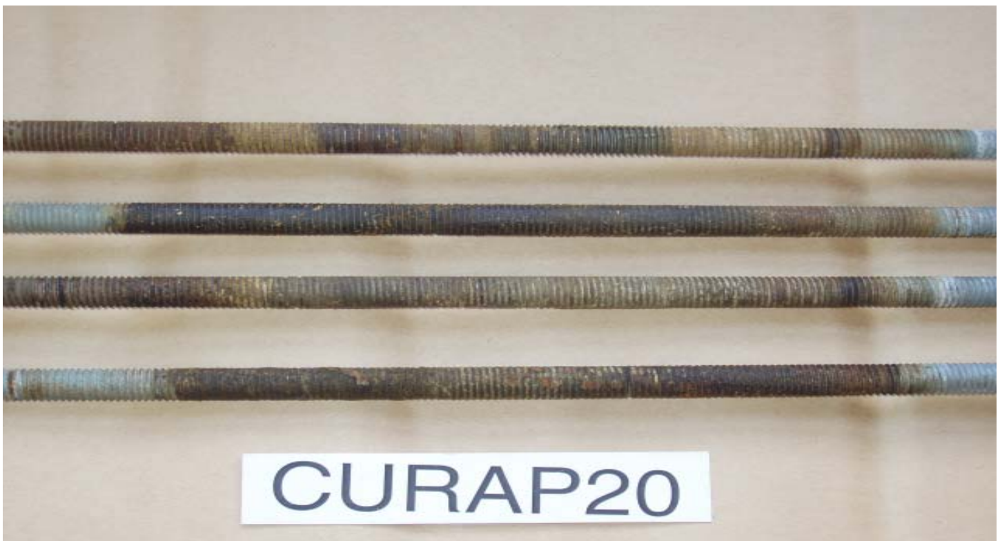
Figure II-2. Condition of CuRap 20 coated galvanized threaded rods after six years exposure in Douglas-fir pentachlorophenol treated pole stubs.
