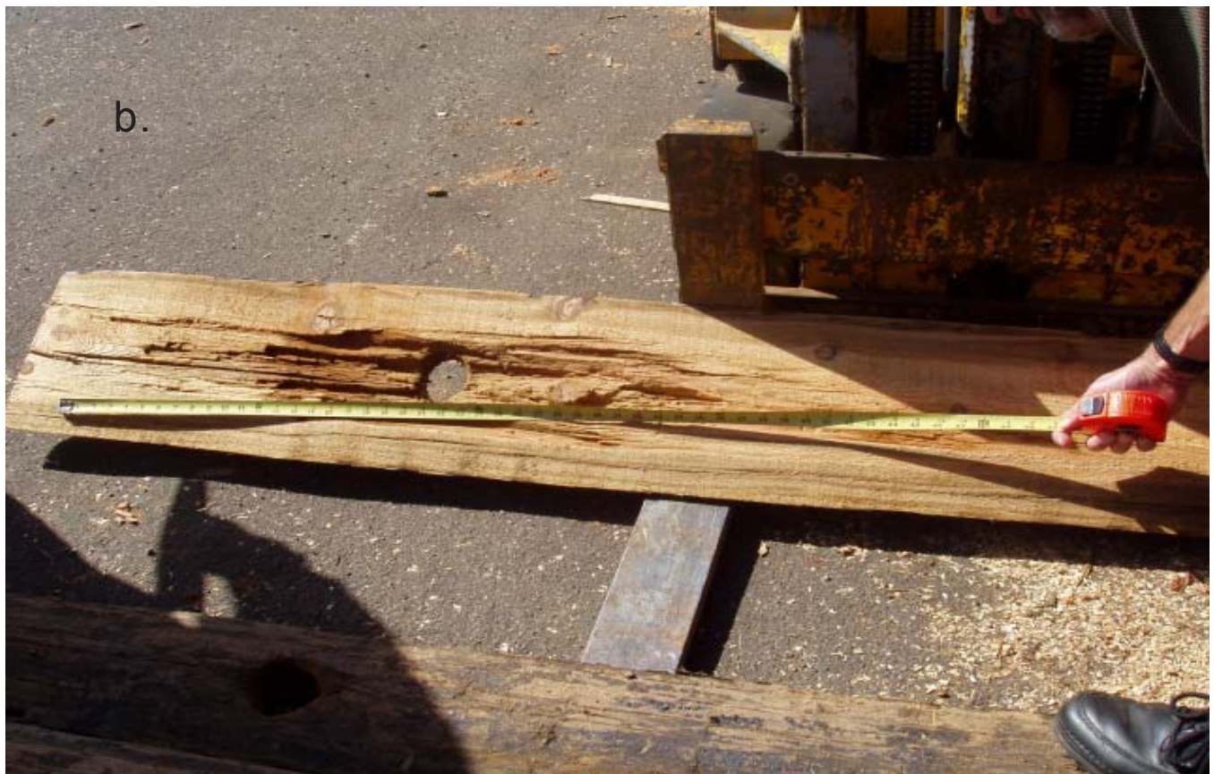
Figure III-4. Example of sections through a Douglas-fir pole showing a woodpecker hole on the surface (a) and the extent of the internal damage associated with the hole (b).
