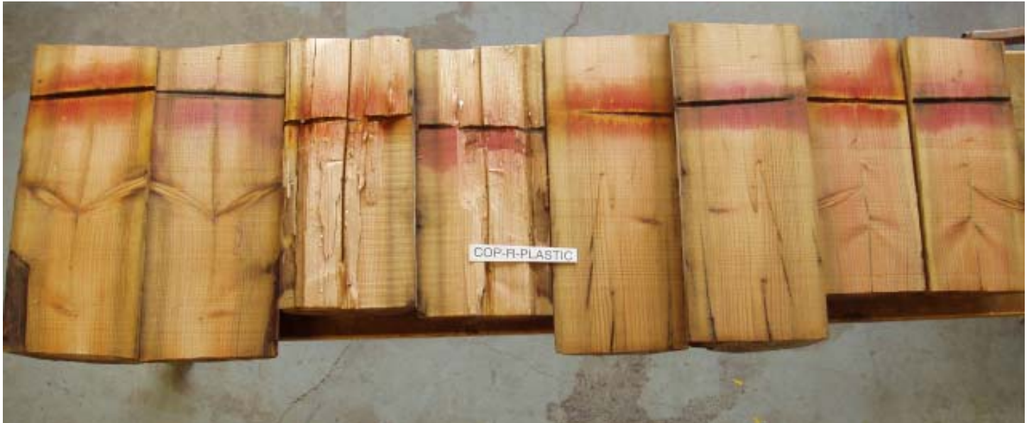
Figure II-3. Degree of copper and fluoride movement away from the sites in Douglas-fir pole stubs where Cop-R-Plastic coated galvanized threaded rods were installed six years earlier. Yellow indicates the presence of fluoride and green-blue indicates the presence of copper.
