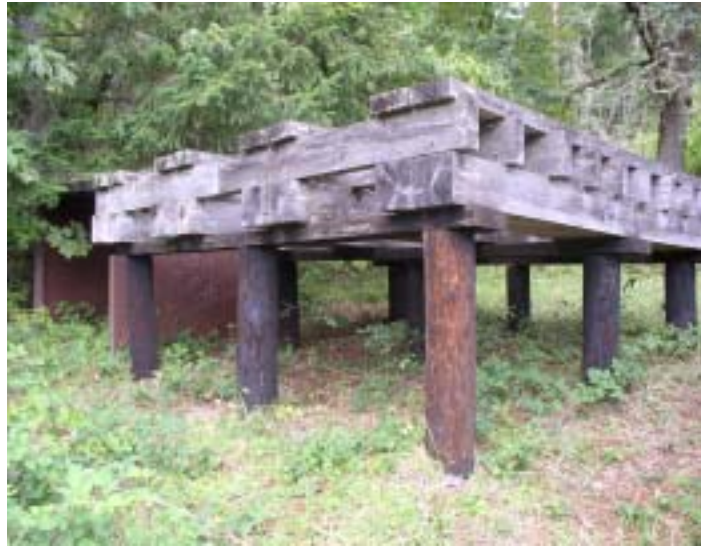
Figure II-4. A simulated pier structure 25 years after construction
