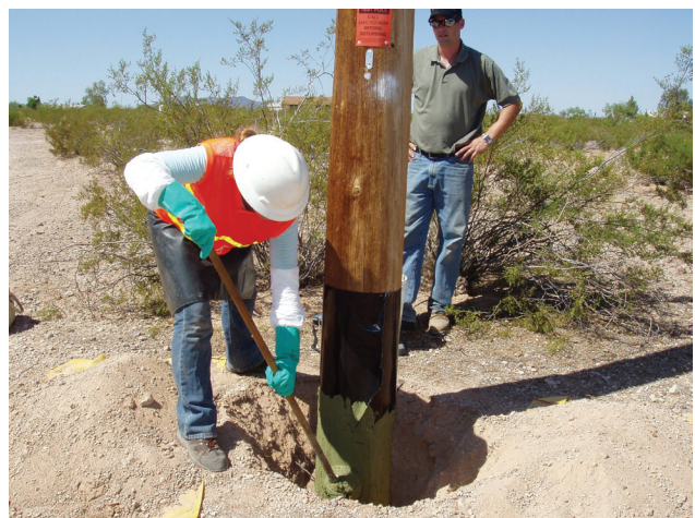
Figure 45. Applying groundline treatment.
