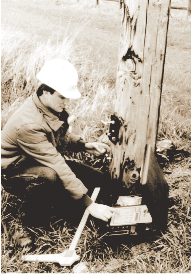
Figure 41. Pole test with an acoustic inspection device.
