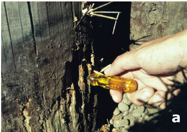
Figure 32. Both external (a) and internal decay (b).
