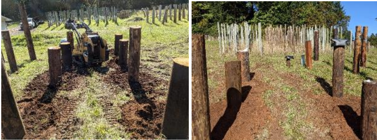
Figure 3.4.1 Peavy Arboretum site for the DCOI pole test.
