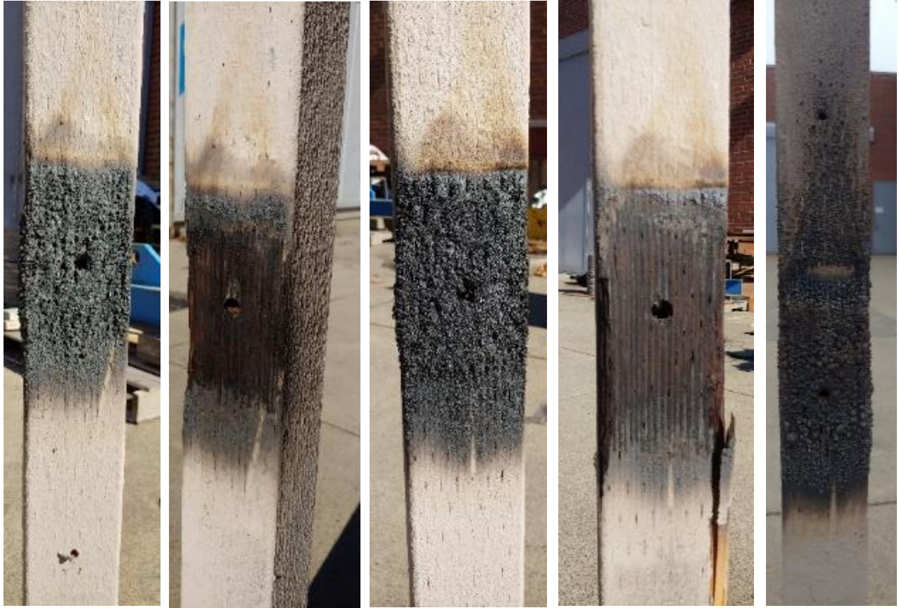
Figure 3.2.7: Coated crossarms after burning with and without remaining char layer from the coating.
