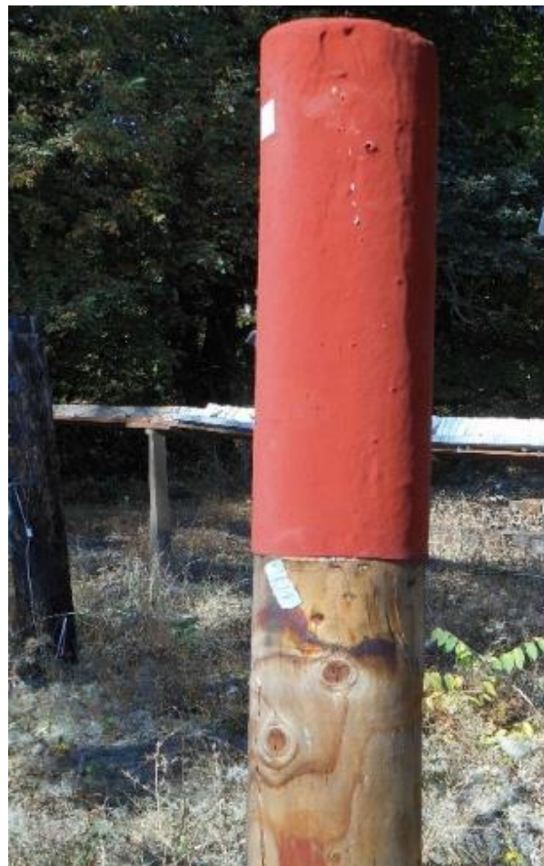
Figure 3.1.2: Example of a polyurea capped pole top during installation in 2011.
